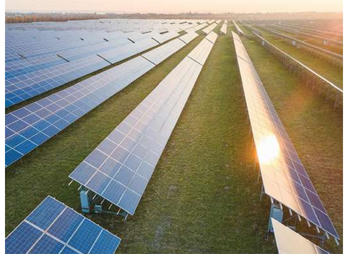
19.50 MWp Type: Ground Mounted Year: 2024 Location: Eastern Africa Status: Under Construction
