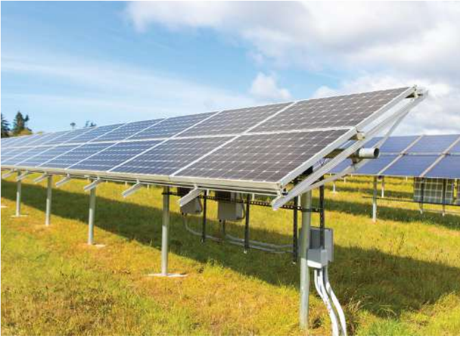
168.00 MWp Type: Ground Mounted Year: 2025 Location: New Zealand Status: Under Construction
