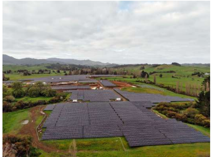
30.70 MWp Type: Ground Mounted Year: 2024 Location: New Zealand Status: Under Construction
