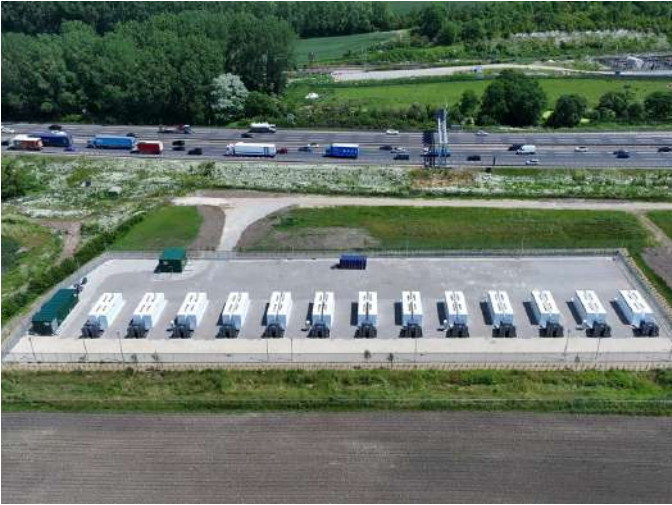
40.70 MWh Type: BESS Year: 2025 Location: Germany Status: Under Construction
